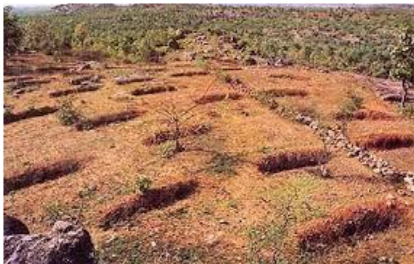
Figure 42: Illustration of staggered trenching Layout
