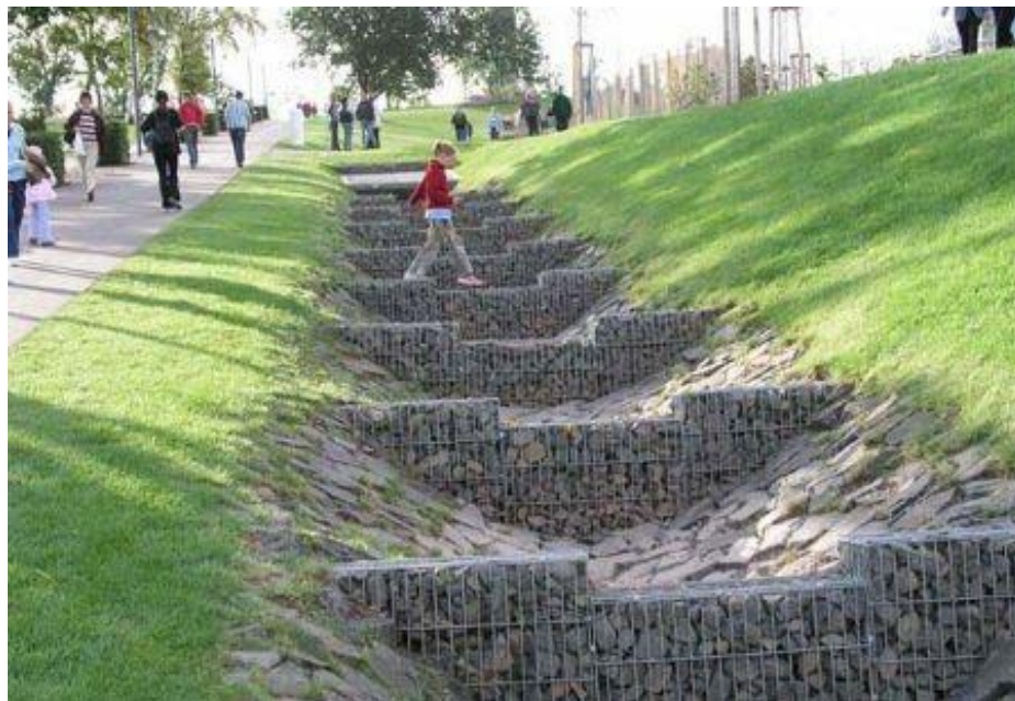
Figure 41: Illustrative diagram of gabion structure
